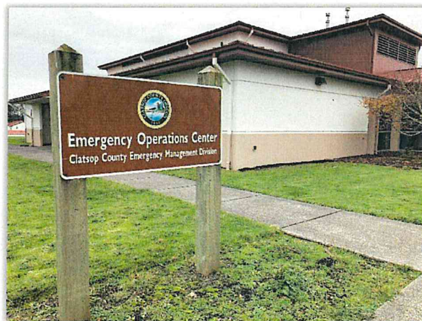
Figure 9: Clatsop County Emergency Operations Center, Warrenton, Oregon
